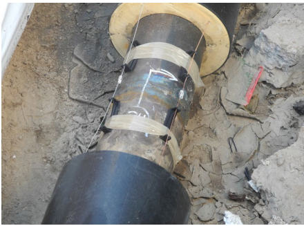
Pre-insulated piping joints connected to controlling conductors (left) and after the mounting of cuffs and foaming
