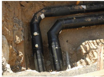
Pre-insulated piping joints connected to controlling conductors (left) and after the mounting of cuffs and foaming
