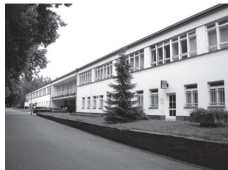
The winner in the "Fire" category was the project pertaining to increasing energy-management efficiency through EPC at the Psychiatric Hospital in Jihlava, Czech Republic
