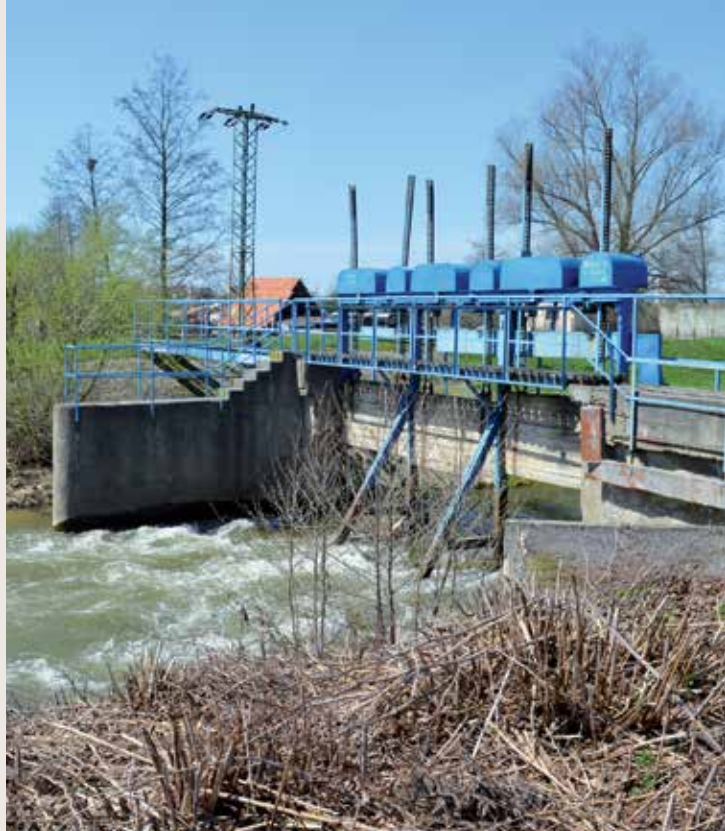
The water gate suitable for installation of a small water turbine | Foto: Poľana-vlnárske závody, s.r.o.
