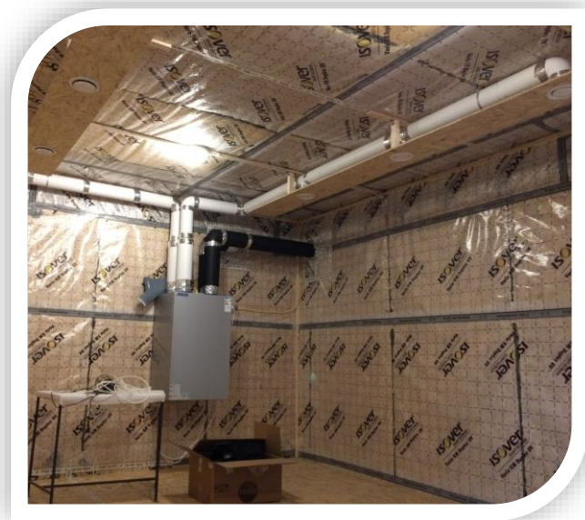
Mechanical Ventilation with Heat Recovery
